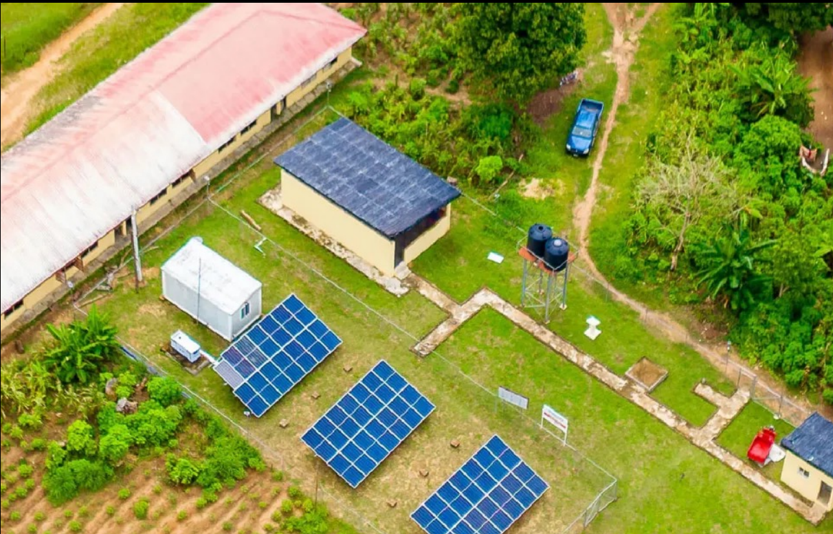
Community solar power facility
